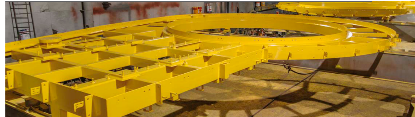
The structure was finally coated with a four-layer paint system from Jotun. The application of each layer required strict supervision as regards conformity with the specified thickness and the requirements of the Norsok m-501 standard.
